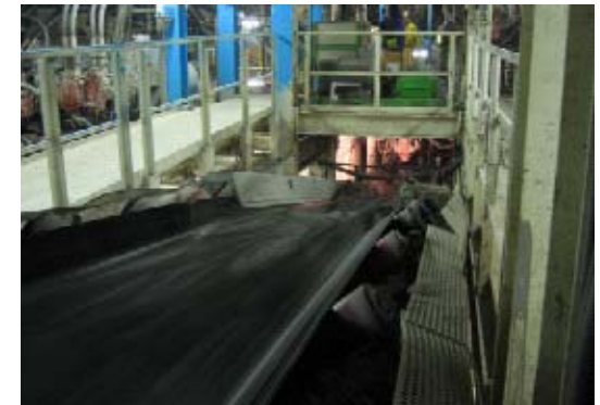
Illus. 6—Excavated material is transported through the rear of the TBM
