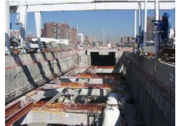
Illus. 5—The TBM launch chamber in Madrid
